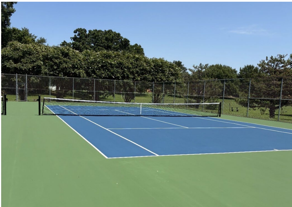
Braden Tennis Court (Project 5)
