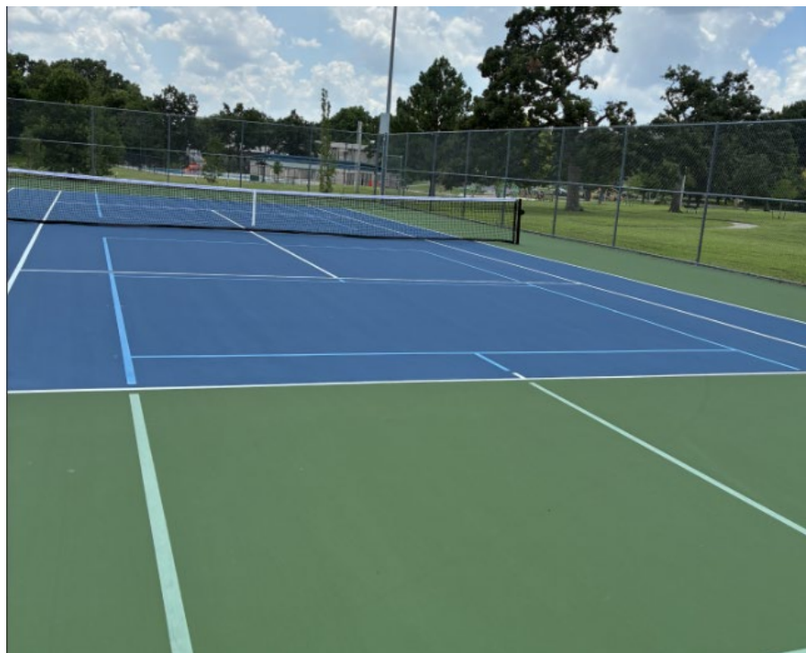
Reed Park Tennis/Pickleball Court (Project 5)
