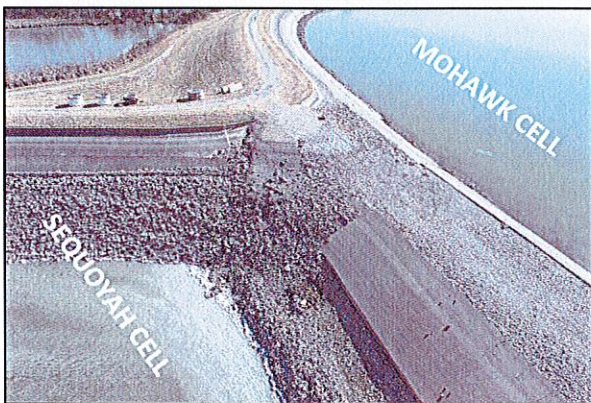
Photo 5 – showing the existing condition of the Sequoyah Boat Ramp project area.
