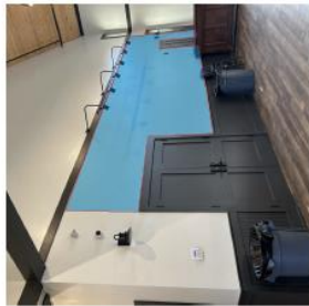
ARRIVAL GALLERY 111 NORTH WALL
