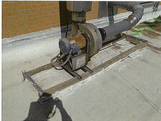
Photo #8 Exhaust fan & support sleepers at Roof 4.
