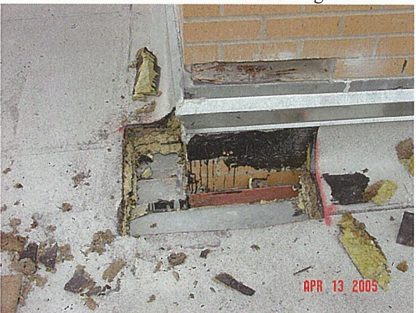
Photo #12 Roof excavation at Area 1.
