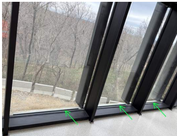
Lights installed along west curtain wall sill.
