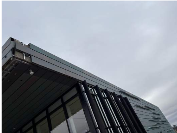
Most coping panels in place around roof edge.
