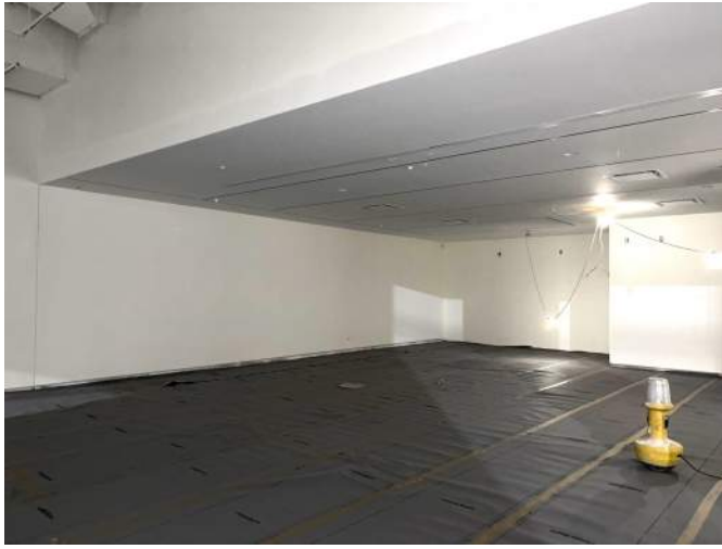
First paint coat applied at L1 East Gallery (poor lighting as power switching to permanent).
