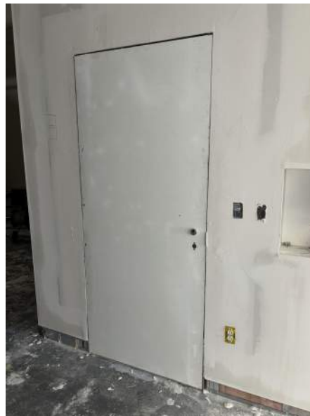
L2 door installations ongoing.
