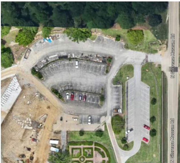
North Parking Lot work begins next week, planned parking changes go into effect.
