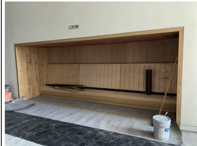
LL2 Benches in place at Elevator 13 Lobby & RR hallway.
