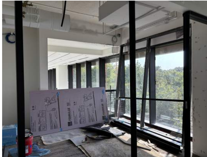
CEO window resizing in progress.
