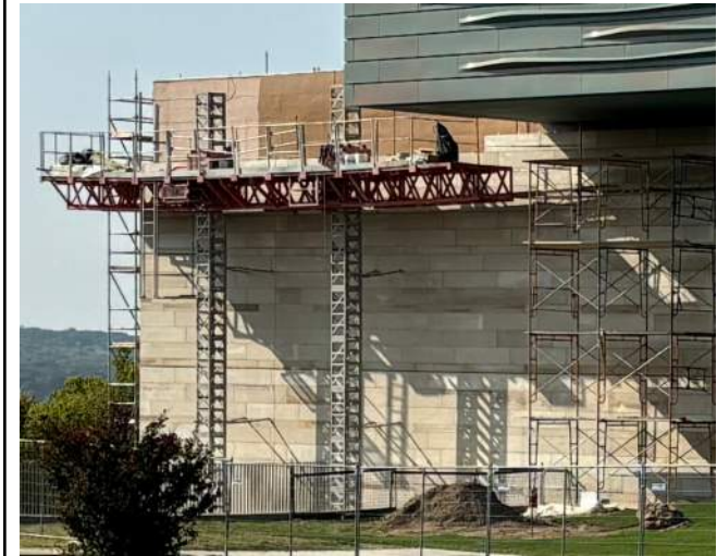
Stone progress continues (Portal stone pictured from interior).
