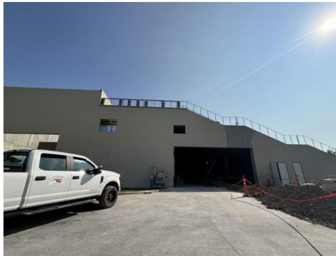
Primer applied at North Amphitheater wall.
