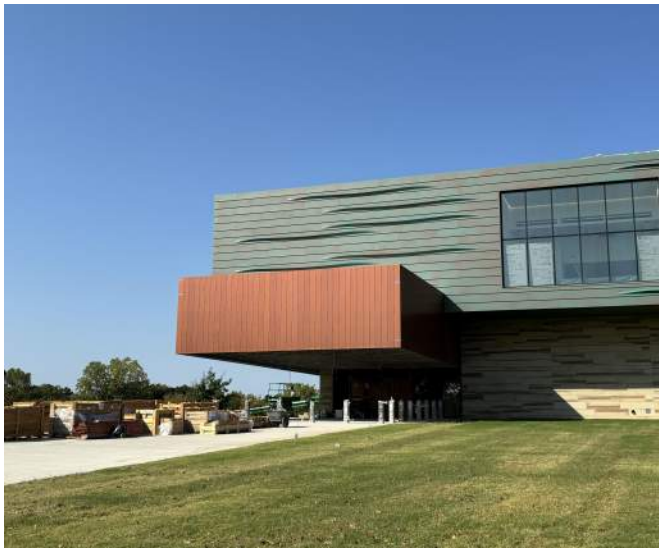
Metal panel progress at Main Entry.
