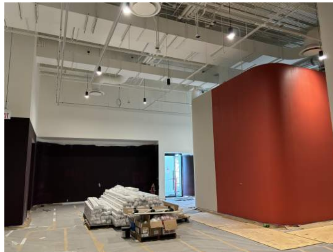
Final paint at LL2 Galleries in progress.
