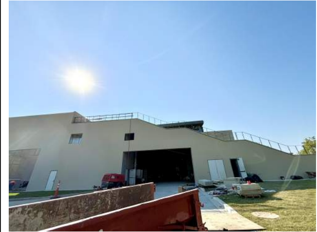
Texture was applied to North Amphitheater wall.
