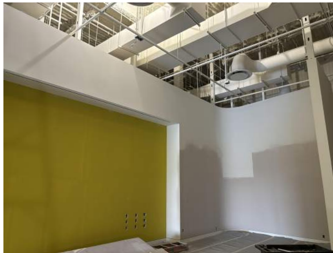
Final paint at L2 Gallery in progress.
