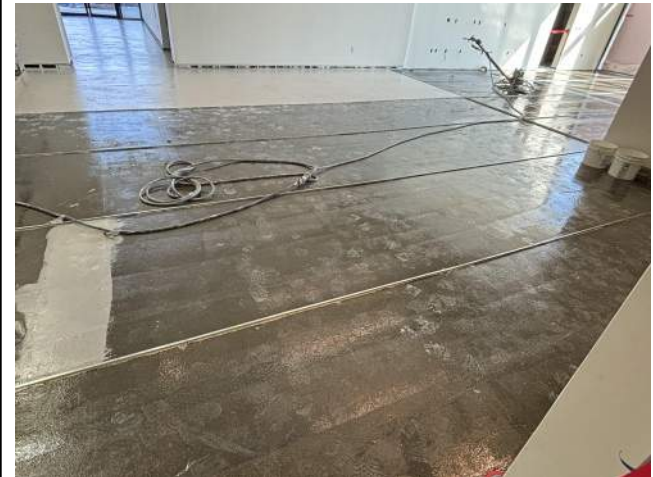
L2 Terrazzo in progress.
