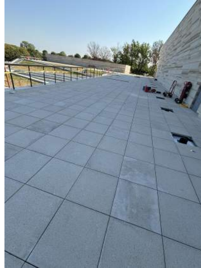
L1 Terrace pavers complete except at drains.
