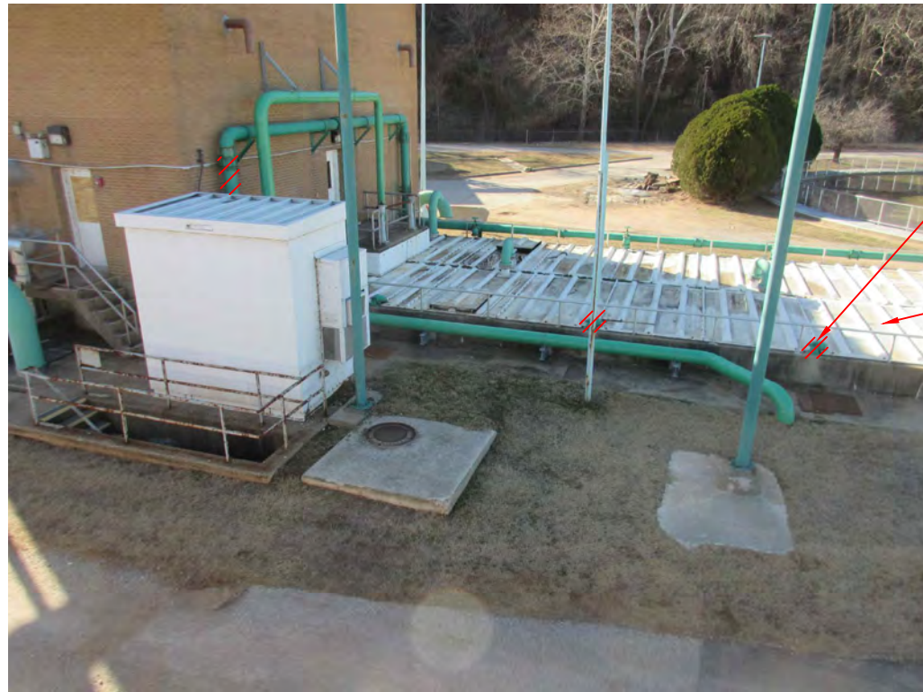
1 PHOTO - BLOWER & ODOR CONTROL PIPING 42 NTS
