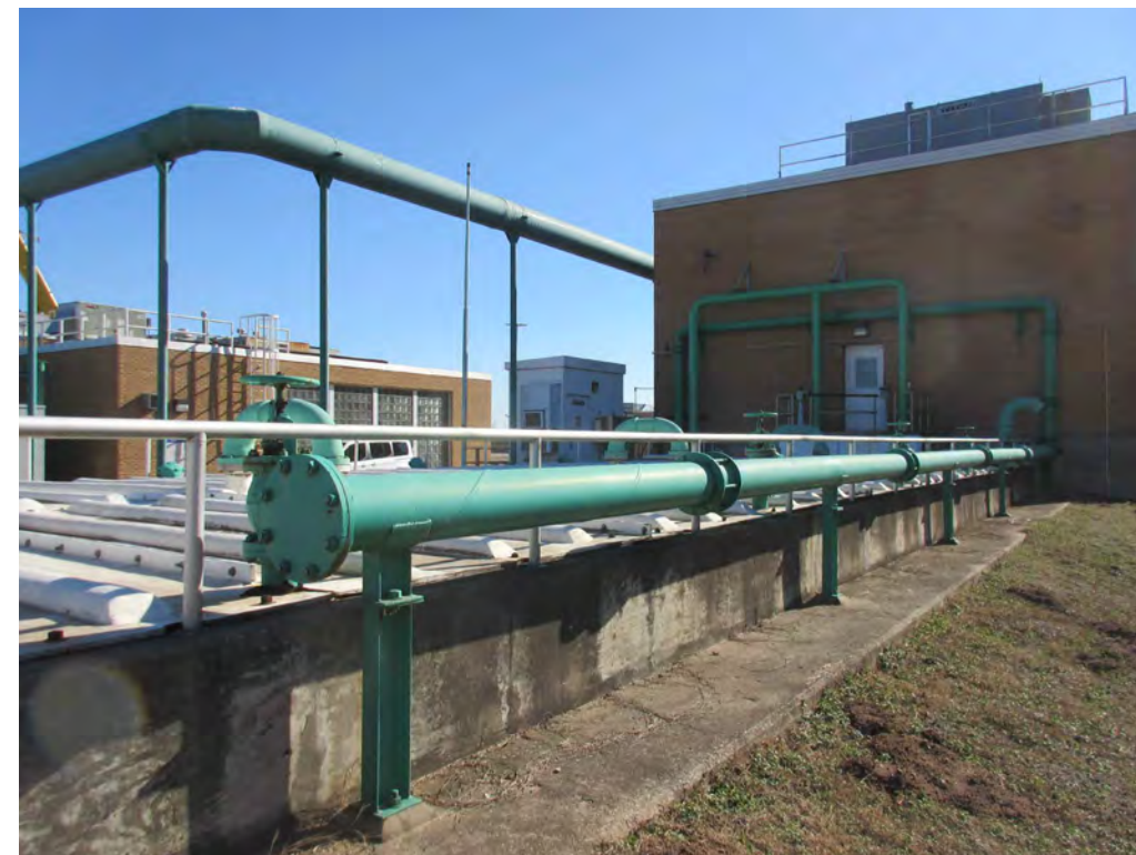
4 PHOTO - BLOWER & ODOR CONTROL PIPING 42 NTS
