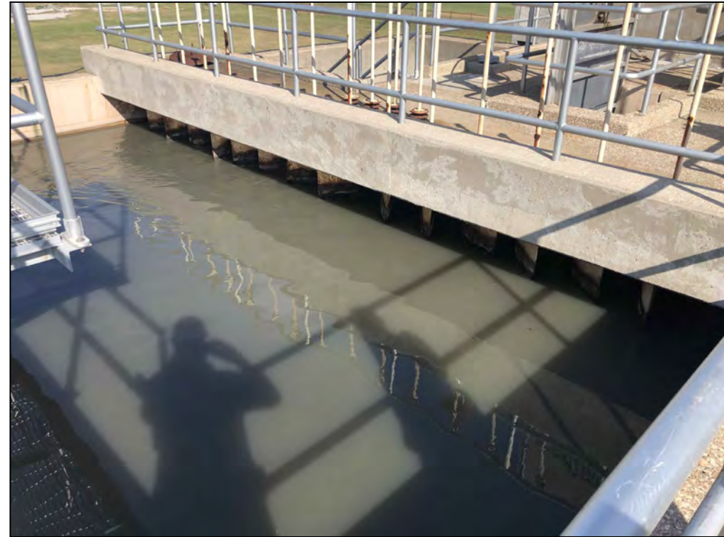
2 6 GRIT COLLECTOR PHOTO SCALE: 3/4" = 1'-0"
