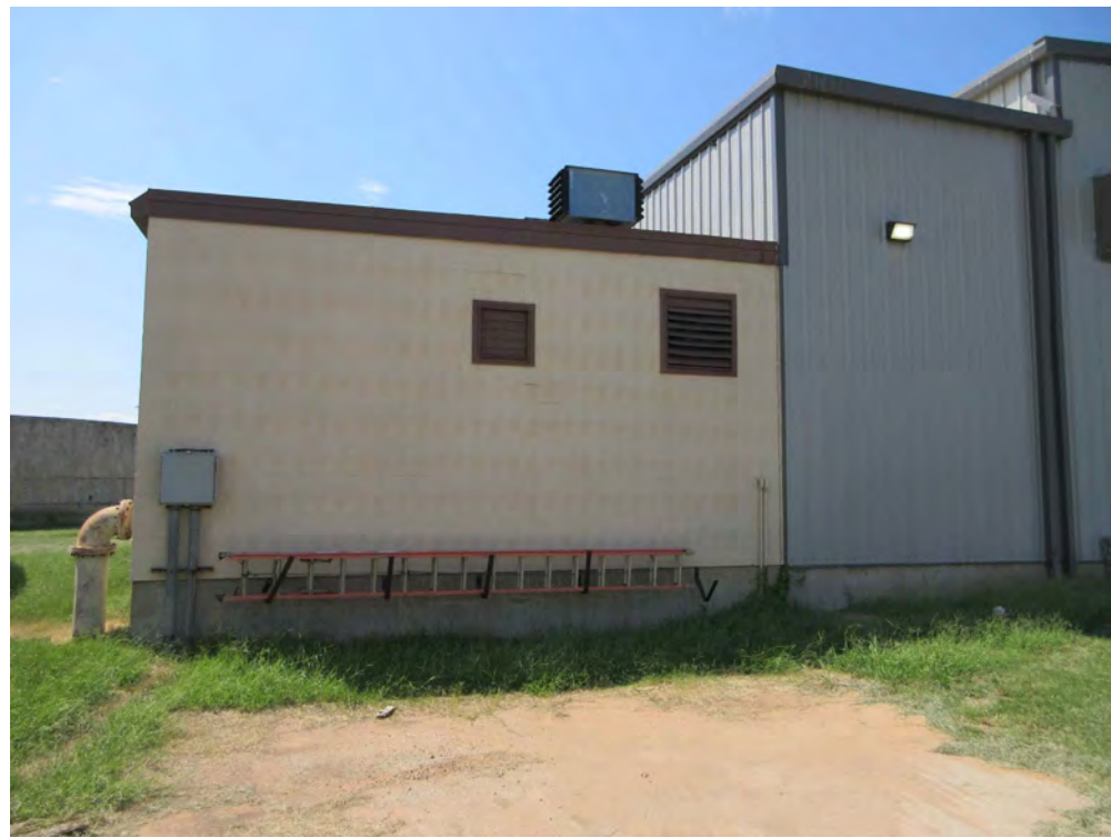
2 MAINTENANCE BUILDING PHOTO 14 SCALE: 3/4" = 1'-0"
